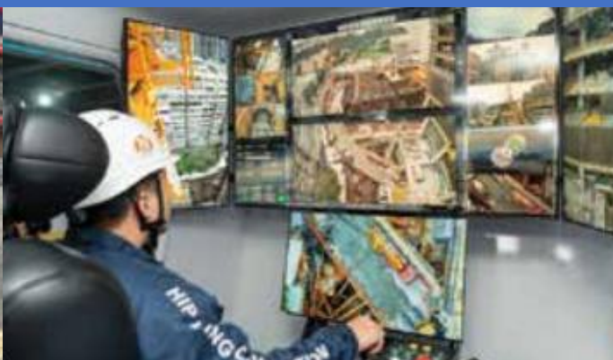
Self-Developed Distant Tower Crane Control System
